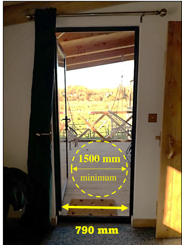
External verandah leading from bedroom 2.
